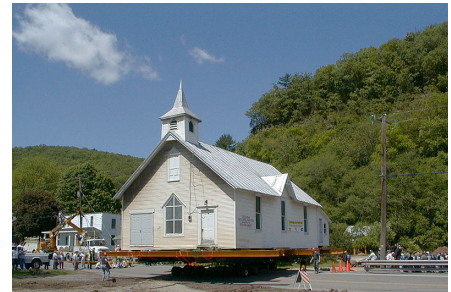
Exhibit 5-2 Small wood frames are the easiest to relocate
