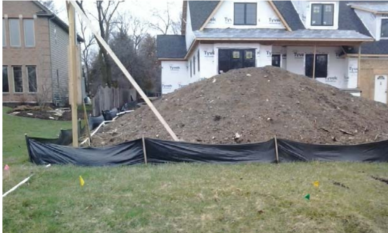
Example of proper erosion control at a new single family development
