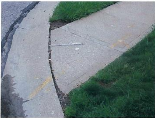
Figure 4L – Low Severity Gap
