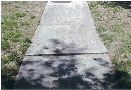
Figure 3L – Faulting 1/2-1"
