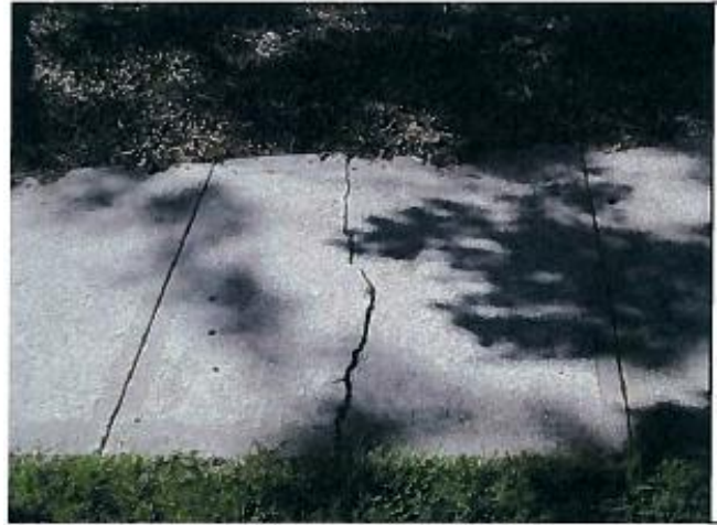
Figure 6L – Low Severity Linear Crack
