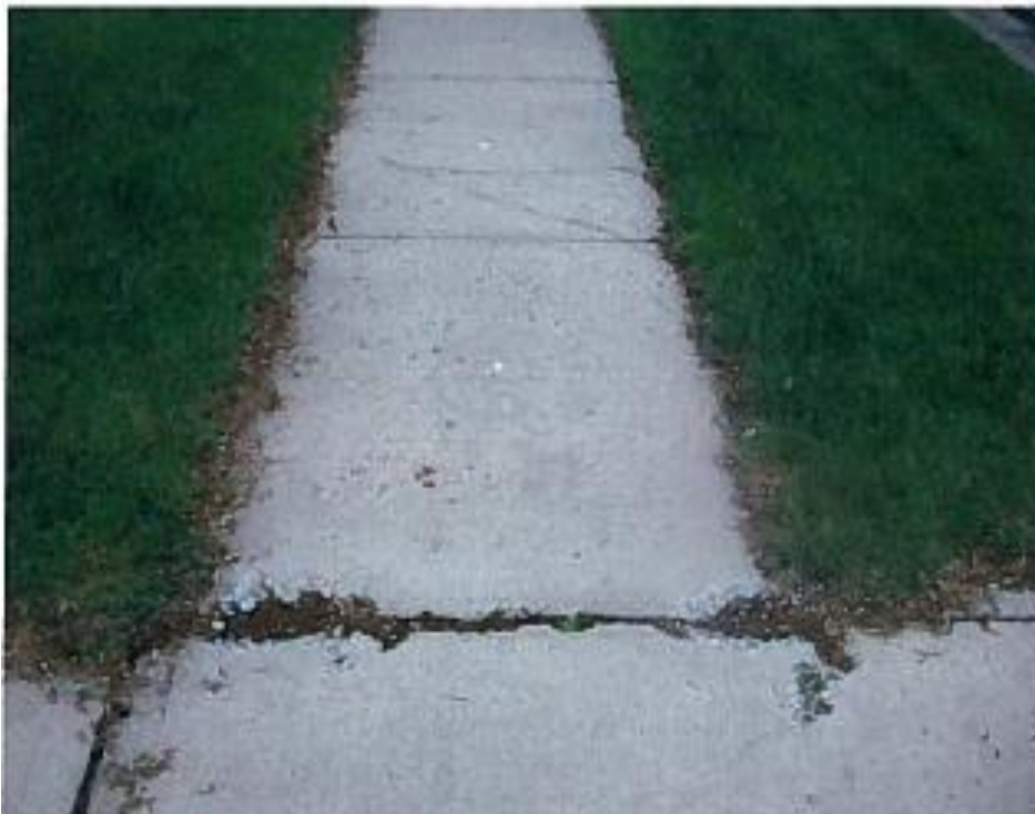
Figure 5L – Low Severity Joint Spalling
