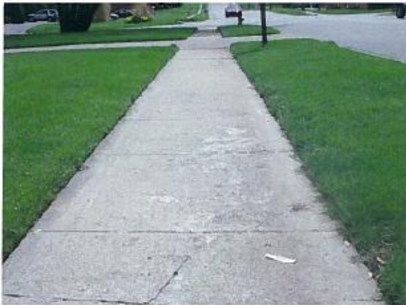
Figure 11L – Low Severity Surface Defects (scaling is present in this photo)
