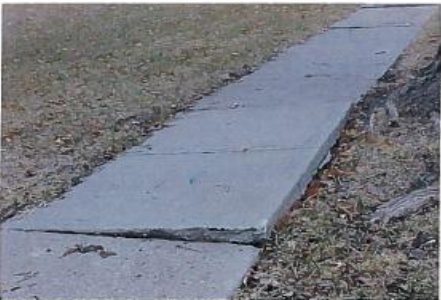
Figure 3H – Faulting >1 1/2"
