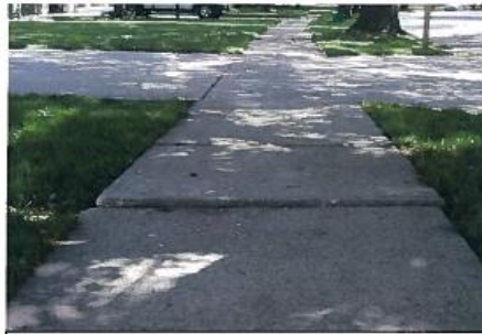
Figure 3M – Faulting 1-1 1/2"
