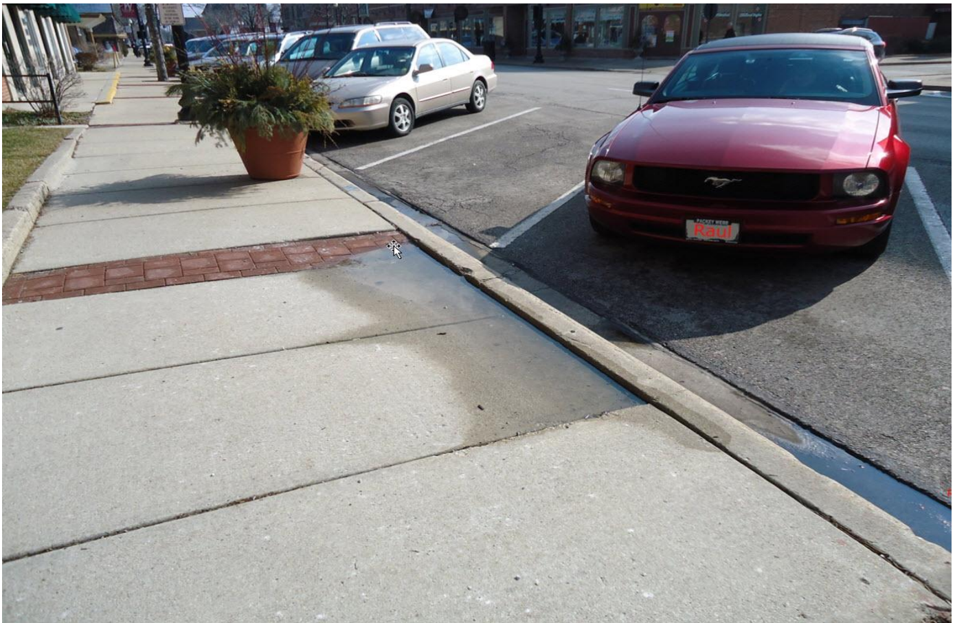
Figure 13 – Longitudinal Faulting Along Curbs
