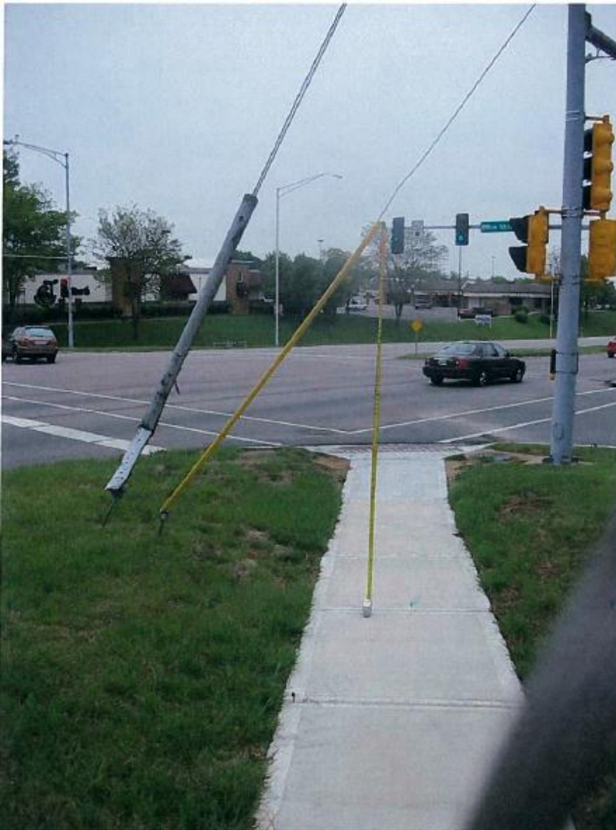
Figure 8 – Protruding Objects (Guy wire is 76" above walk)
