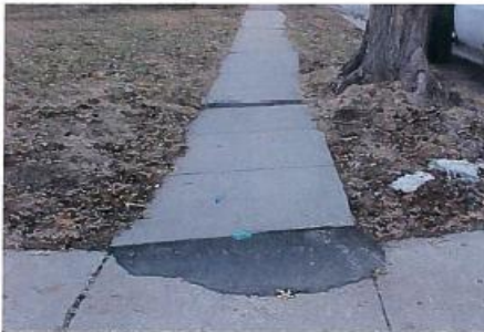
Figure 3P – Patched Fault
