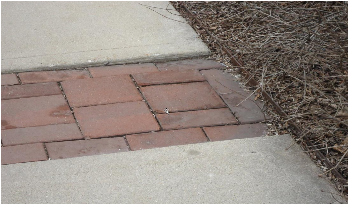
Figure 12 – Paver Brick Settlement
