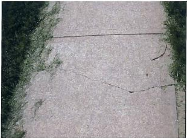
Figure 6N – Non-faulted Linear crack
