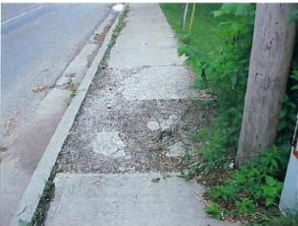
Figure 11H – High Severity Surface Defects
