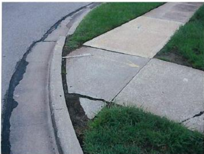
Figure 4H– High Severity Gap
