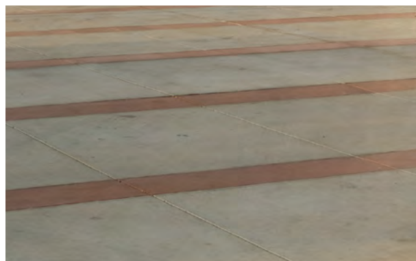
Sidewalk Alternative - Scored Concrete with Colored Bands
