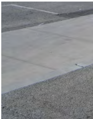
Porous Pavement or Porous Concrete (in parking areas)
