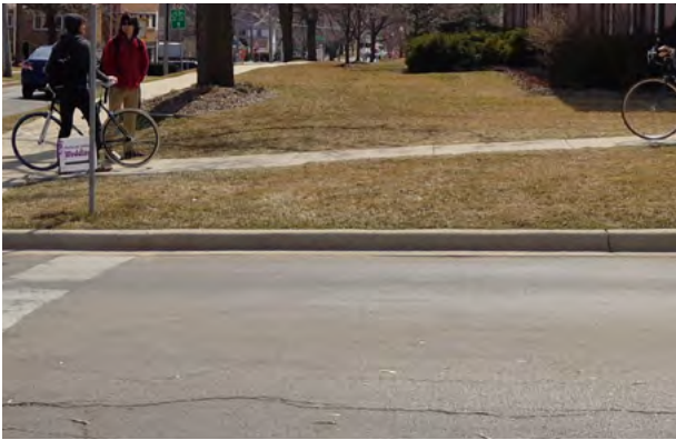
Typical Concrete 6" Curb Treatment
