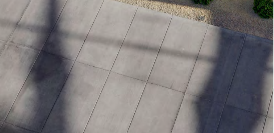
CONCRETE SIDEWALK WITH DESIGNED JOINTING PATTERN
