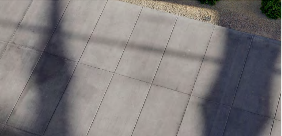
CONCRETE SIDEWALK WITH DESIGNED JOINTING PATTERN
