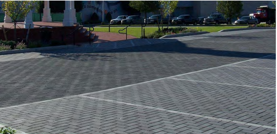
PERMEABLE PAVERS OVER PERCOLATING BASE Unilock Eco-Priora pavers
