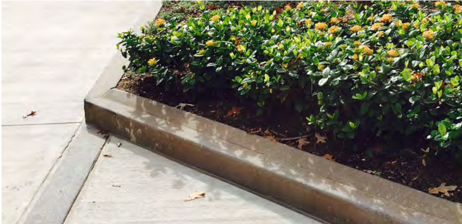
6" CONCRETE CURB WITH A DESIGNED PROFILE
