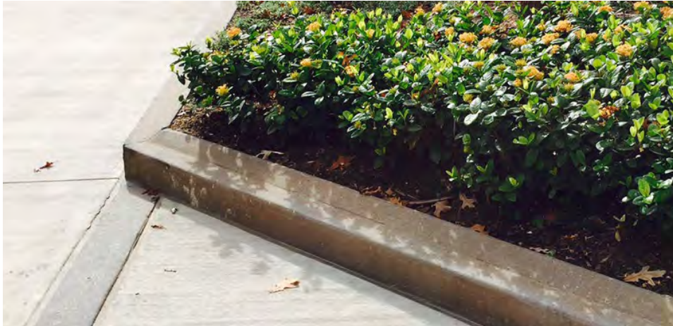
6" CONCRETE CURB WITH A DESIGNED PROFILE
