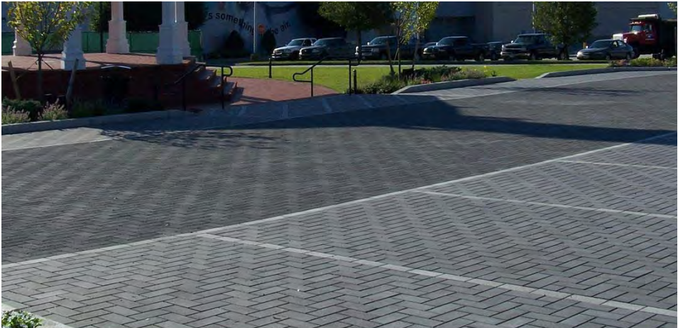
PERMEABLE PAVERS OVER PERCOLATING BASE UNDER ENTIRE ROAD Unilock Eco-Priora pavers
