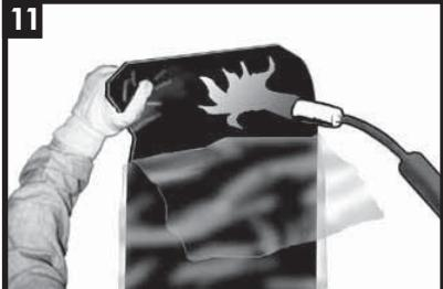
Partially remove the release liner and gently heat the underlap approximately 150 mm (6") from the edge.
