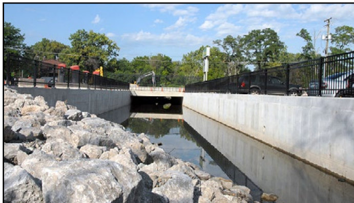
The North Main Street Flood Control Project has included widening the creek channel that runs under Main Street.
