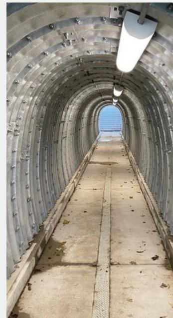
The pedestrian tunnel under Roosevelt Road at Wheaton Avenue is now open! Crews lined the existing tunnel ceiling and walls with metal plates, replaced the lighting and handrails, and poured new concrete flooring and stairs. The City had previously closed the tunnel due to deteriorating materials in the decades-old passageway under Roosevelt Road.
