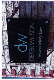
1 METAL SIGNAGE PLATE ON STAND OFFS WITH INTERNALLY ILLUMINATED SIGNAGE AT ALL TENANTS
