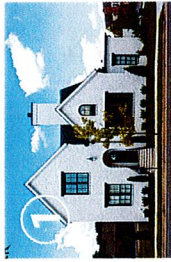
WHITE STAIN APPLIED TO PORTIONS OF CENTER WITH GABLE AND HIP ROOFS WITH GREY STAIN ON BRICK DETAILING
