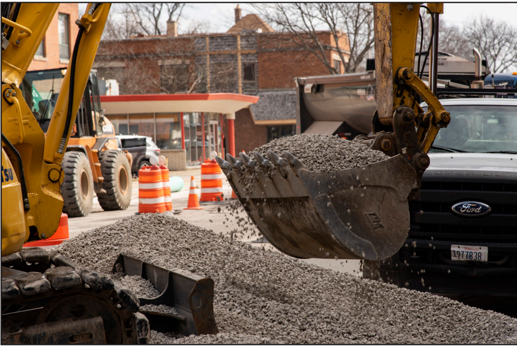
Crews are digging to replace storm sewers on Wesley Street as part of the project.
