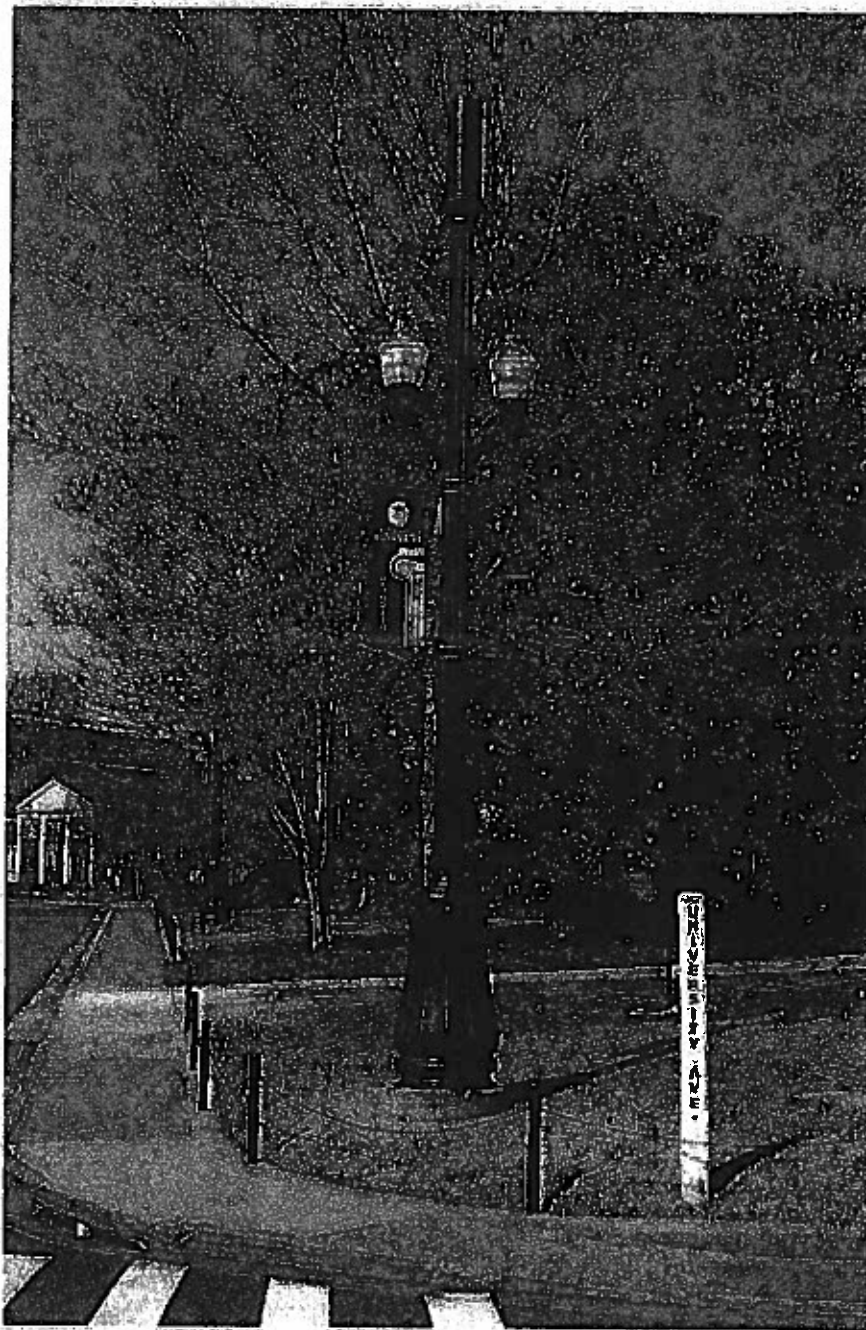
Exhibit 5. This design may be acceptable if consistent with other fixtures in the immediate vicinity. The base is out of scale to the arms and luminaires. In addition, while symmetrical, the pole and antenna extend far above the luminaires, making the design appear vertically out of proportion. Arms and luminaires should be within the top 20% of the pole height. This design is prohibited; however, a similar design may be acceptable with appropriate modifications.
