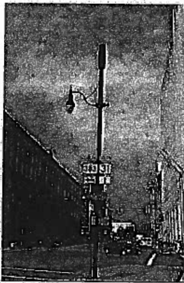
Exhibit 12. The pole lacks a base in scale to the volume of the antenna, which is larger than the diameter of the pole and does not appear to be an original part of the pole. This design would be prohibited.
