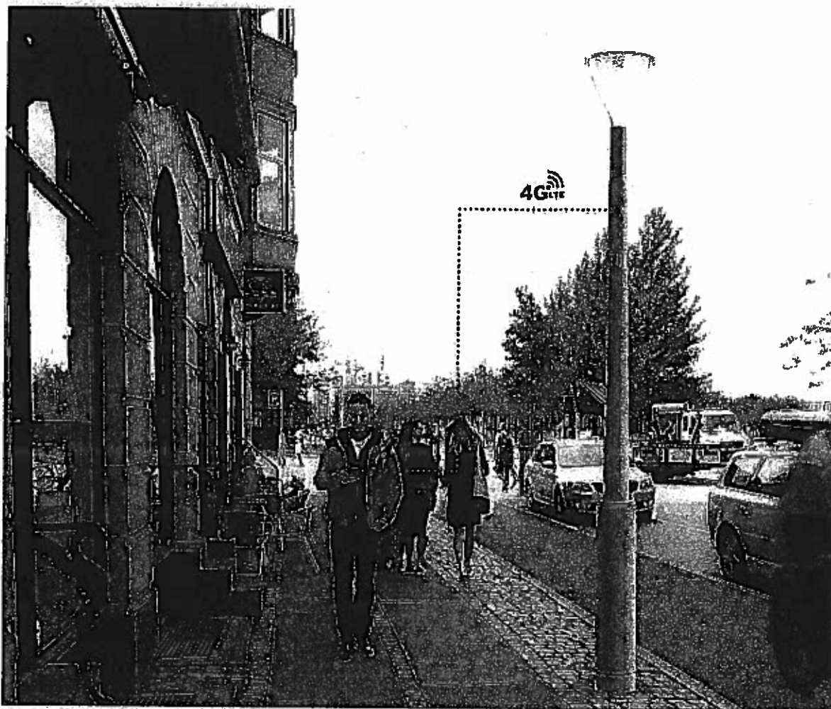
Exhibit 3. An antenna incorporated into, and hidden in the pole of top mounted, pedestrian scaled light may be acceptable if painted black, featured an acorn luminaire, and otherwise substantially resembled the acorn light fixtures already existing in the City. The photo depicts a Philips pole with internal Ericsson antennas.
