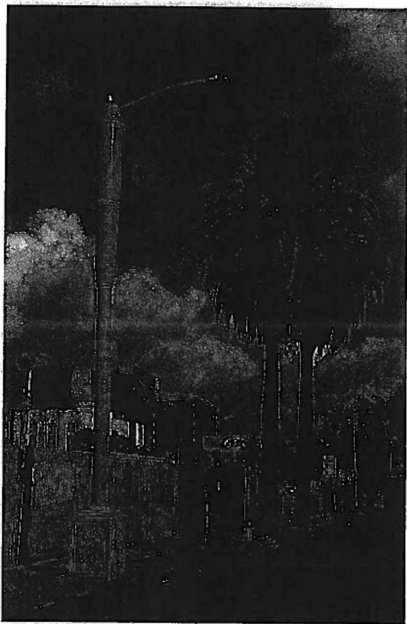
Exhibit 7. The antenna enclosure has a larger diameter than the pole, rendering it insufficiently cloaked. This design is prohibited.
